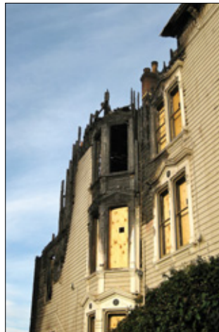
A three-flat Victorian on Golden Gate was badly damaged.
